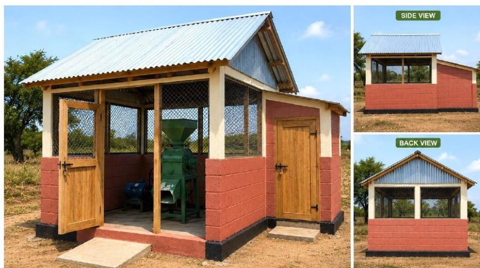
Fig2: A sample picture of a semi-permanent grain mill shelter with small attached storage space for small-scale business
