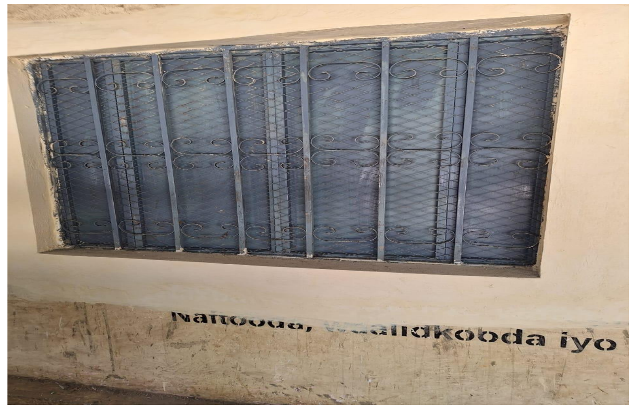
Front side view, steel windows
