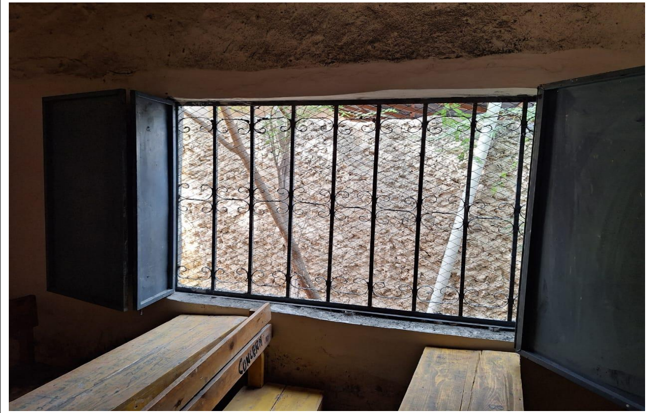
Rear view steel windows
