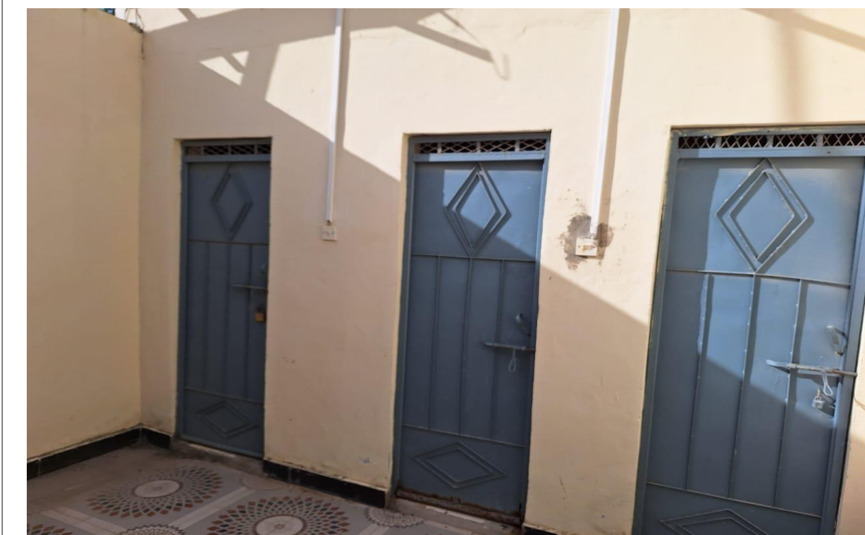
Front view, for rehab VIP toilets, male Teachers.
