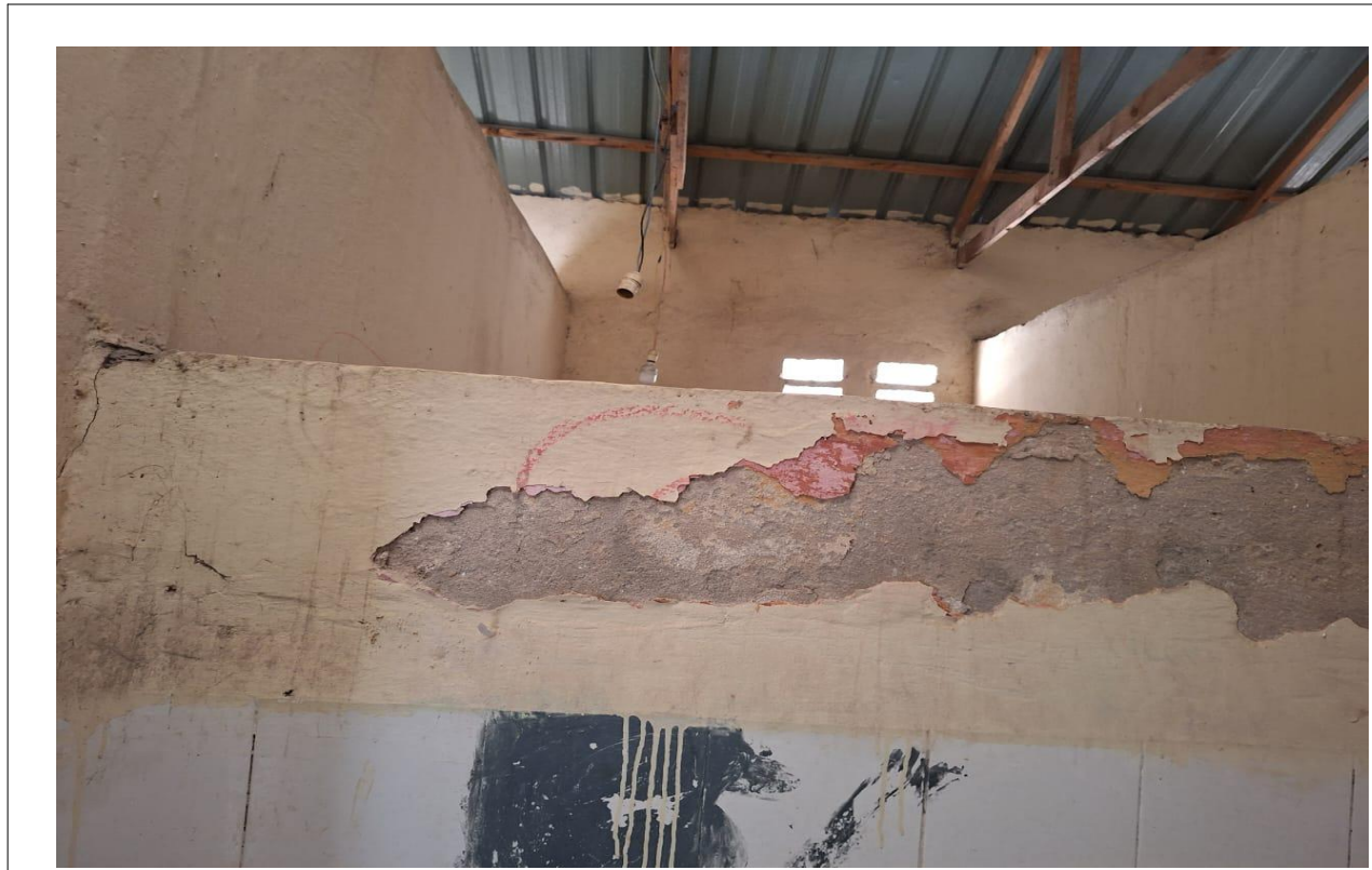
Inside view, rehab for boys toilets
